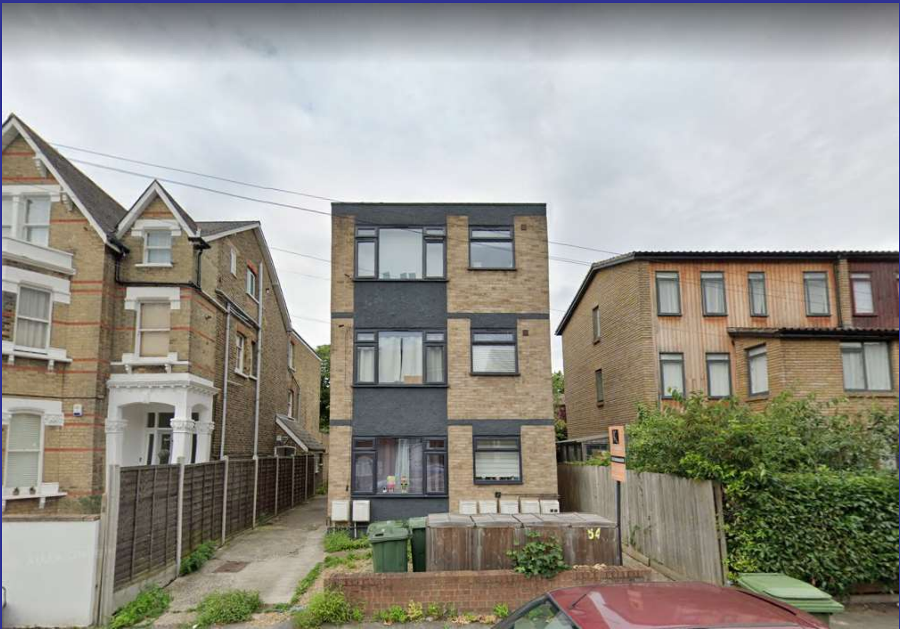
Existing three storey property
